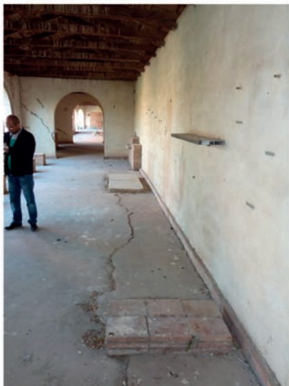
Fig. 27. Archaeological Area of Apollonia: a) theater, effect of lanslide phenomena along the western flank of the acropolis; b) collapse of the walls in the acropolis; c) fractures relate to the instability phenomena inside the monastery and church of the Saint Mary; d) Effect of gravity sliding on the eastern wall.
