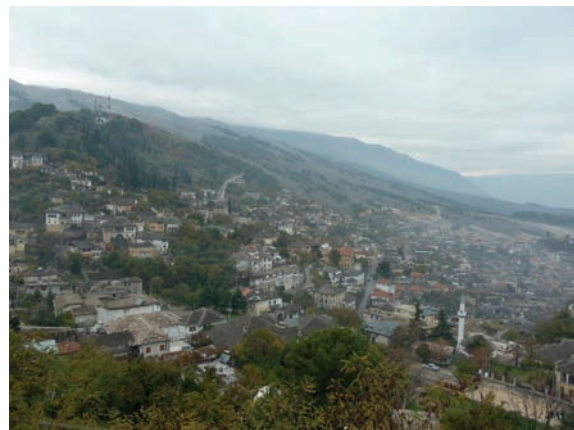
Fig. 51. View of Gjirokastra from the southwestern hilltops of the city. In 1965, the historical monuments were declared under protection of the Institute of Monuments. The area was supervised by experts of the field in harmony with the directives of Venice Charter.
