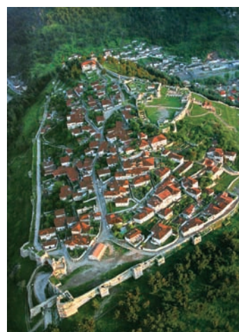
Fig. 33. Aerial view of the Berat fortifications.
