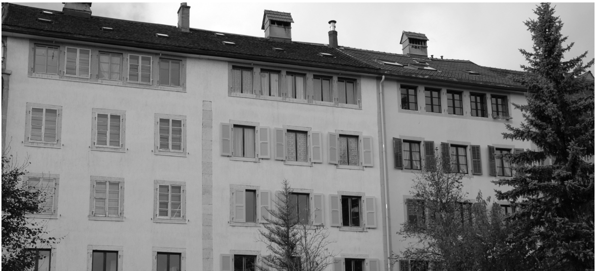
Working class housing, mid 19 th century - La Chaux-de-Fonds
