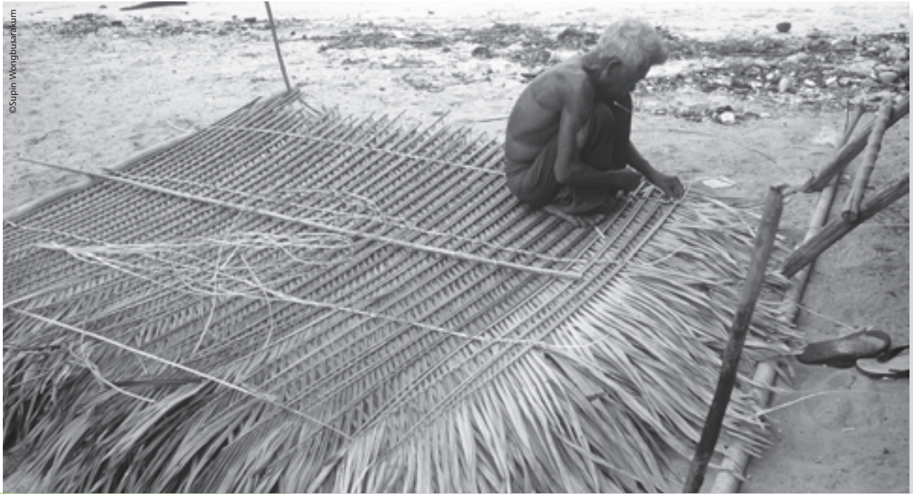
Making a roof from rattan and nipa palm
