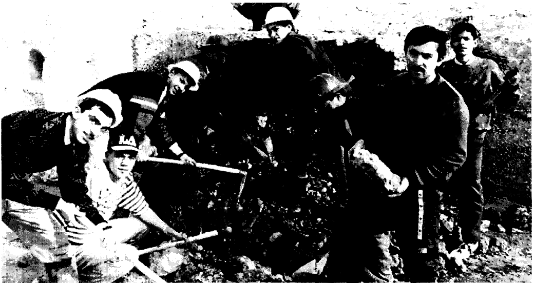
Restoration work in the Medina of Fez (Morocco), organized by the World Federation. Photo WFUCA and UNESCO Centre of Khémisset.
