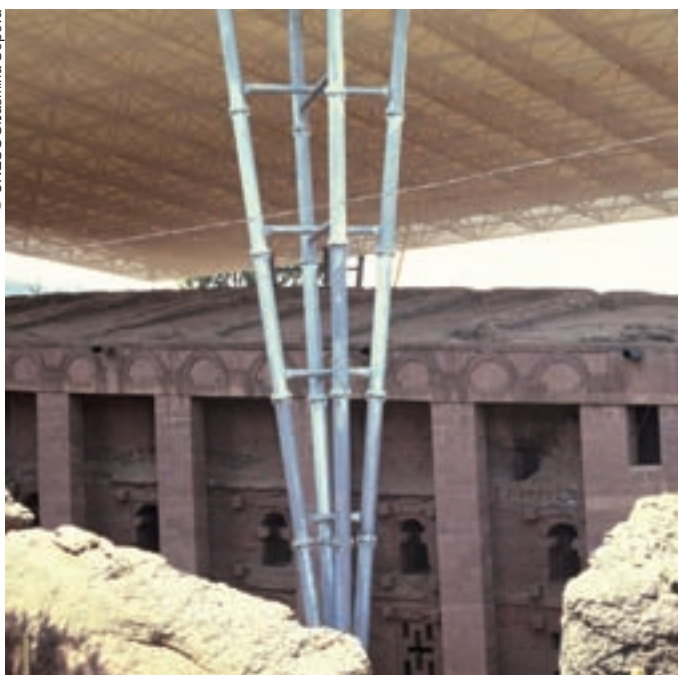
Beta Medhane Alem, the largest church in Lalibela, under a modern shelter.
