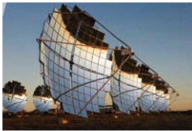
Solar array at Lajamanu, Northern Territory © DEWHA/ Dragi Markovic
