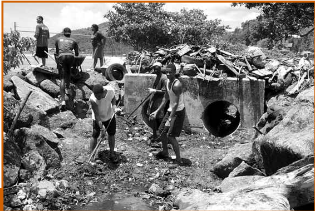
Students and community members clearing the blocked drain.
