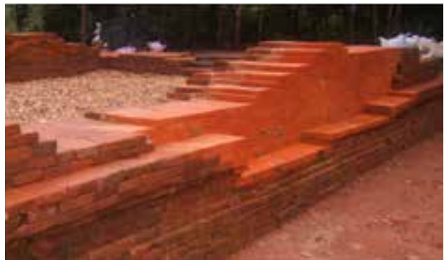
The wall of G3 was reconstructed using the anastylosis
