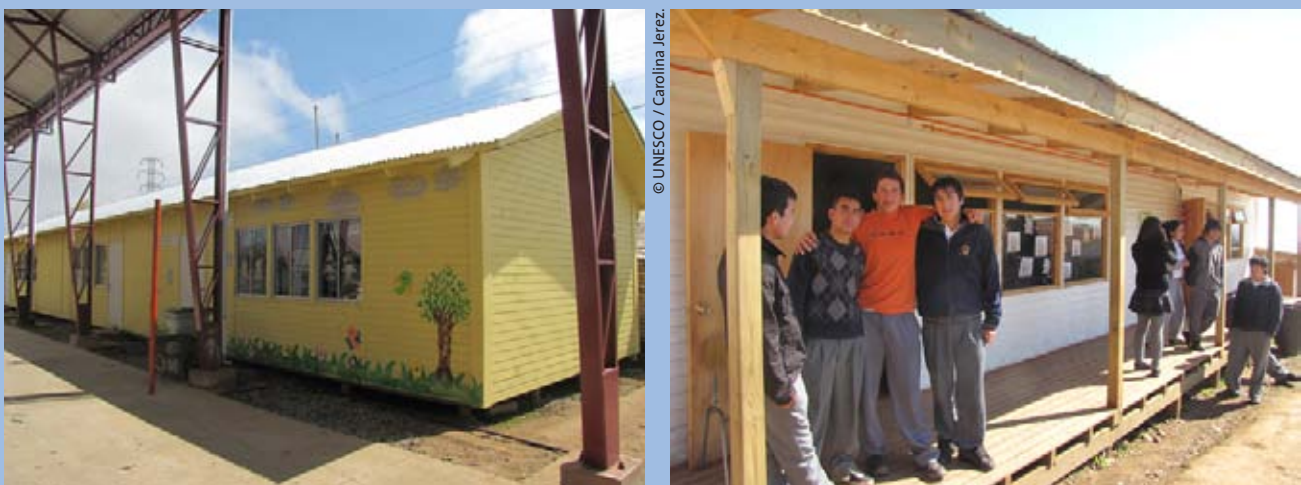
Views of temporary learning spaces constructed by UNESCO to provide emergency education in the most affected areas of the country.
