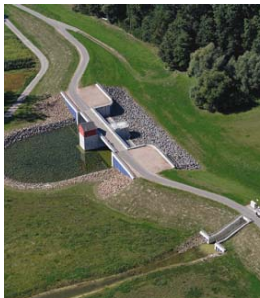
The works in the Polder Ingelheim, north of Mainz in Germany
