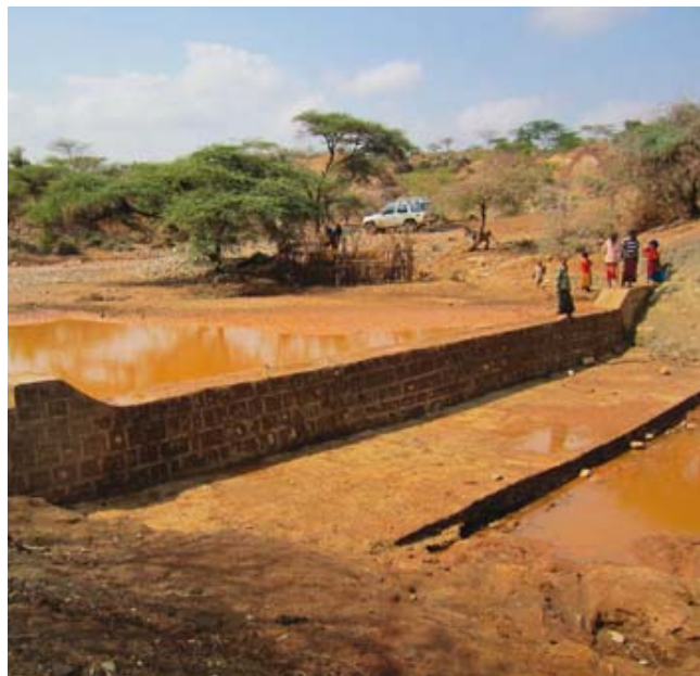
A sand dam in East Ethiopia which creates enough groundwater to supply the nomadic population and its cattle with safe water the whole year through
