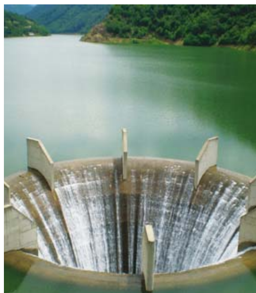
A spillway on the Prvonek Dam in Southern Serbia
