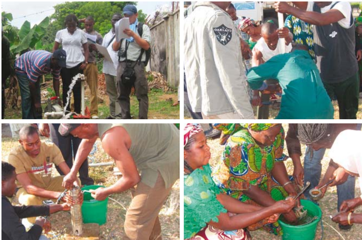
A Youth Empowerment Programme field demonstration. Clockwise from top left: borehole pumping test; dismantling a submersible pump; women service the submersible pump; coupling the serviced pump before reinstallation
