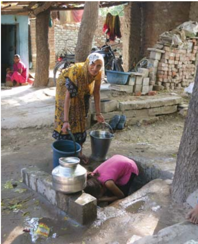
A community water post in a slum community in Ahmedabad, India; the community set the tap below ground level to improve water pressure
