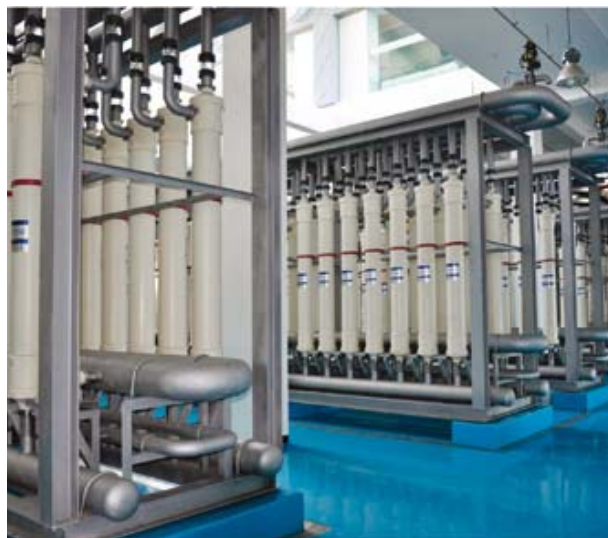
Yeongdeungpo waterworks: the DIMS pressured membrane (left) and HTM submerged membrane (right)
