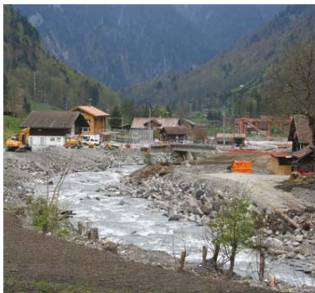
River regulation works in the Lütschine basin in Switzerland
