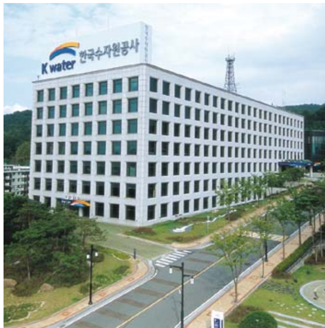
The headquarters of the Korea Water Resources Corporation (K-water)
