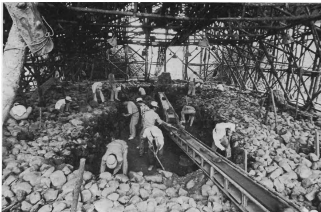
The stones are removed beneath a temporary structure erected to protect the site.
