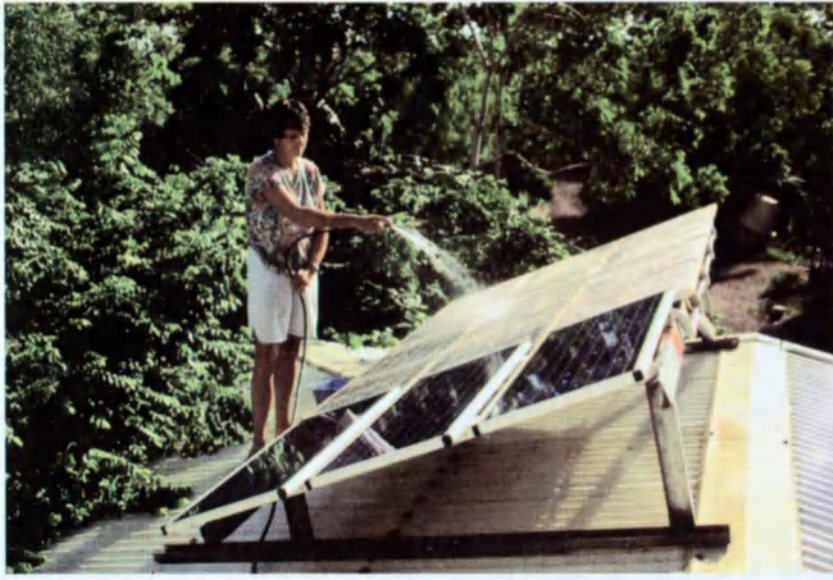
C leaning domestic solar heating panels in Australia.
