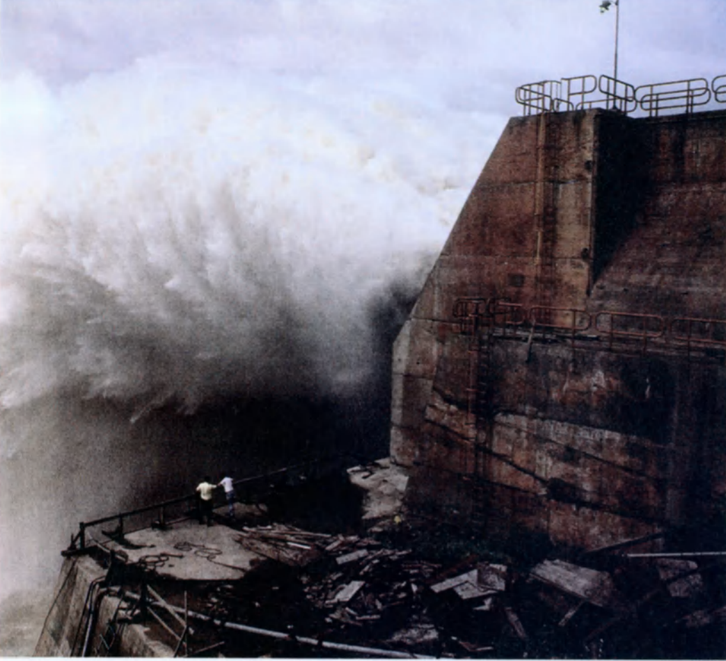
Itaipu dam on the Parana river (Brazil and Paraguay).
