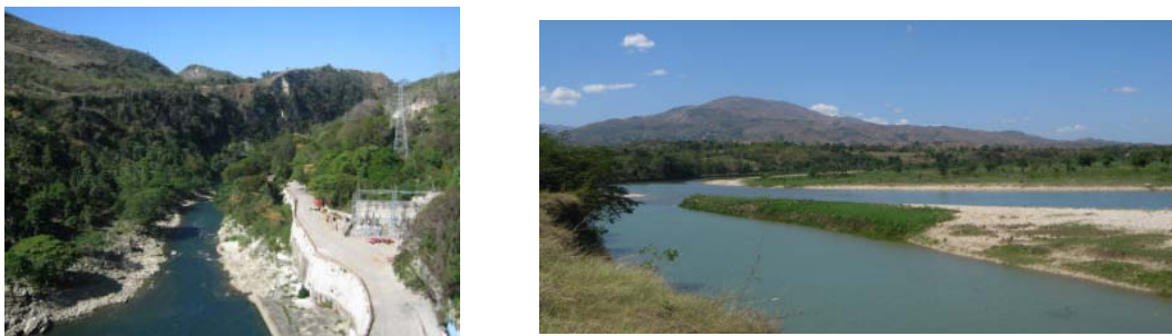
Figure 8: Artibonite River (at Peligre Dam, and between Mirebalais and Canneau)
