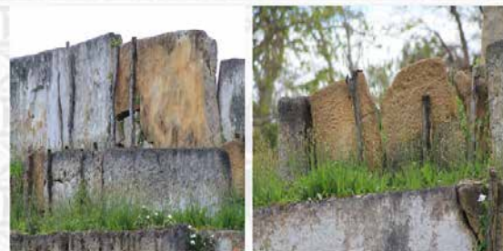
Fig. 4: Conservation works to stabilize facing stones on the langi at Lapaha.
