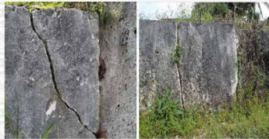
Fig. 3: Impact of previous earthquakes on the Site. The Sites contains huge stone slaps - some pieces weight over 20 tons.
