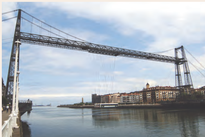
Vizcaya Bridge (Spain)
