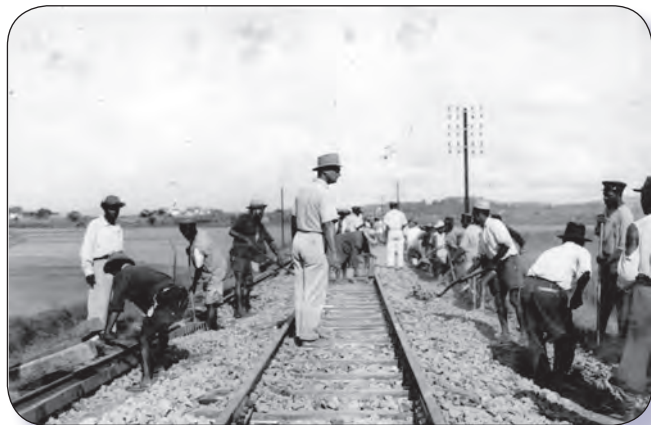
Forced labour for the construction of the railways: tamping ballast under the sleepers.
