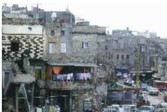
Detail of the seafront façade of the Old City of Saida. After the Israeli bombardment in 1982, refugees moved into the Old City, constructing over Ottoman-epoch buildings
