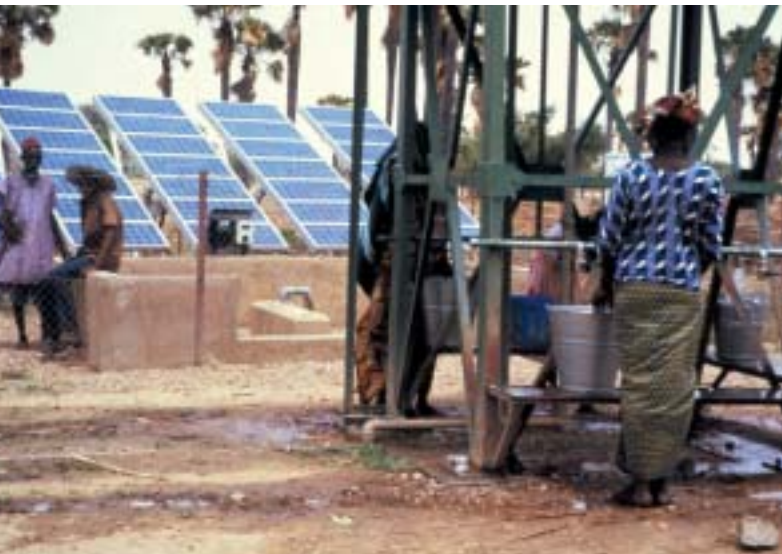
Collecting buckets of water from a solar-powered pumping station. This saves village women and girls from having to walk several kilometres each day to fetch water
