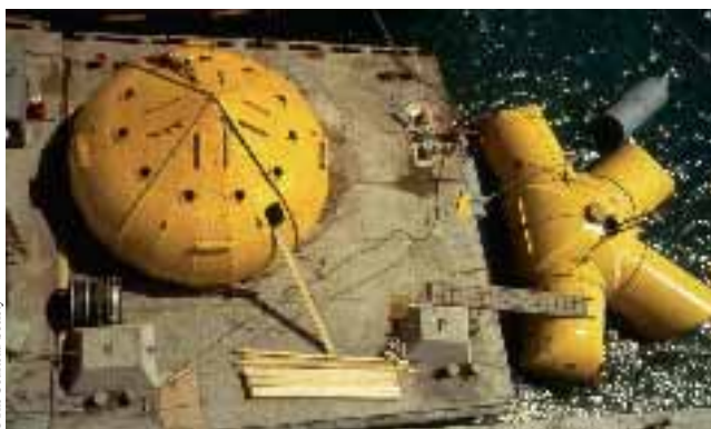
The Conshelf II village is assembled on the surface before being submerged. The oceanauts' star-shaped house is in the water, ready to be sunk to a depth of 10 m. On the quay, the bathyscaphe hangar has just been completed
