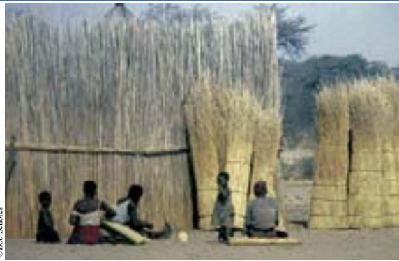
Reeds being dried in preparation for use in construction, in the Caprivi region of northern Namibia
