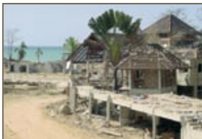
Destroyed tourist resort at Khao Lak in Phang Nga Province, Thailand. Homes and hotels constructed in places not traditionally inhabited were often the most exposed and the most extensively damaged
