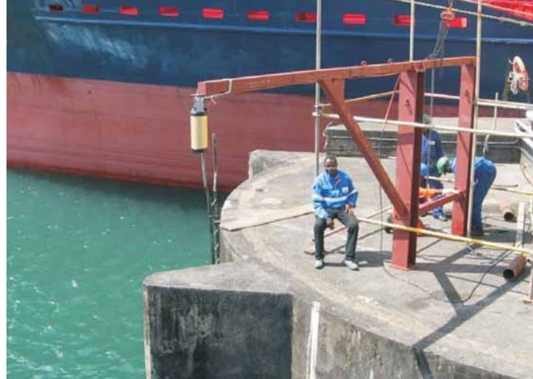
Figure 5. Tide gauge installed at Port SONARA (photo credit: Frédéric Simon, 22 June 2008).
