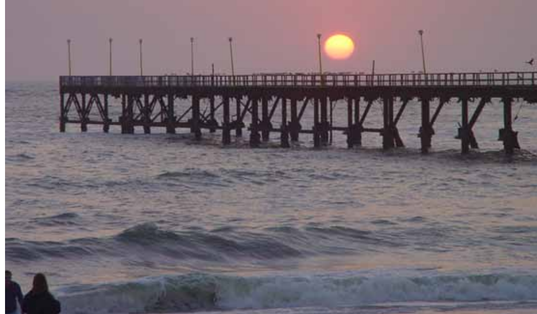
Figure 1. Jetty in Swakopmund where measuring equipment are attached for daily water samples for temperature, oxygen and phytoplankton (photo taken by Deon Louw).
