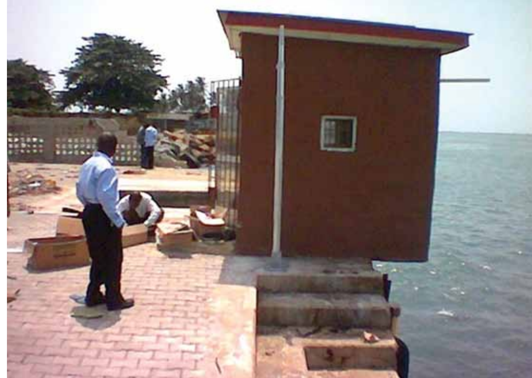
Figure 3. Lagos tide gauge house.
