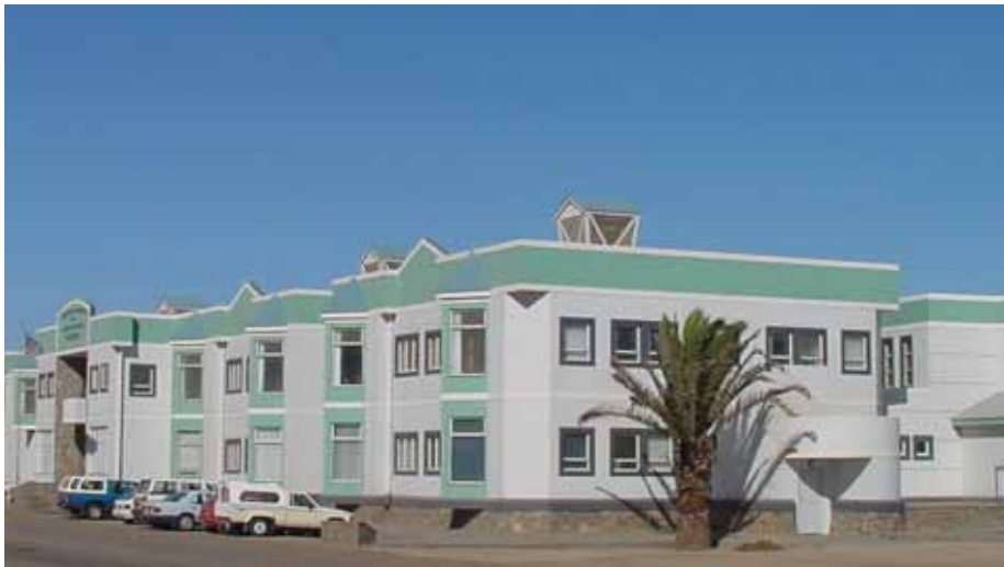
Figure 5. NatMIRC (National Marine Information and Research Centre) offices in Swakopmund. The National Aquarium as well as the following research section are situated here: Environment, Demersal, Pelagic and Aquaculture (Mariculture) (photo taken by Deon Louw).
