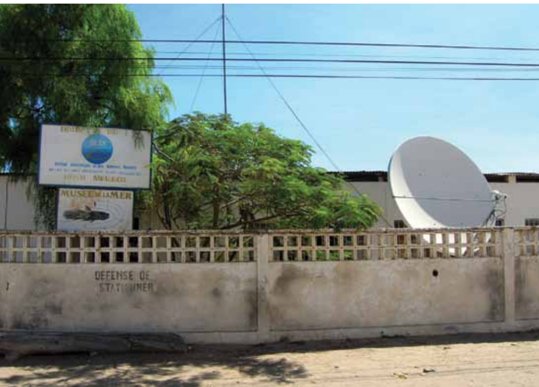
Figure 2. Satellite dish for VSAT link installed at IHSM with ODINAFRICA support.
