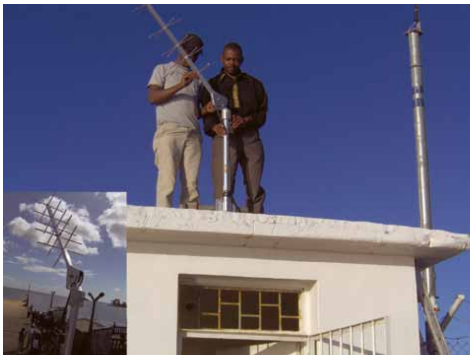
Figure 1. The GPS antenna installed in Inhambane Tide Gauge station.
