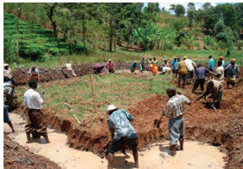
Photo 6: Community participation in constructing a fish pond for Thuita Forest Network
