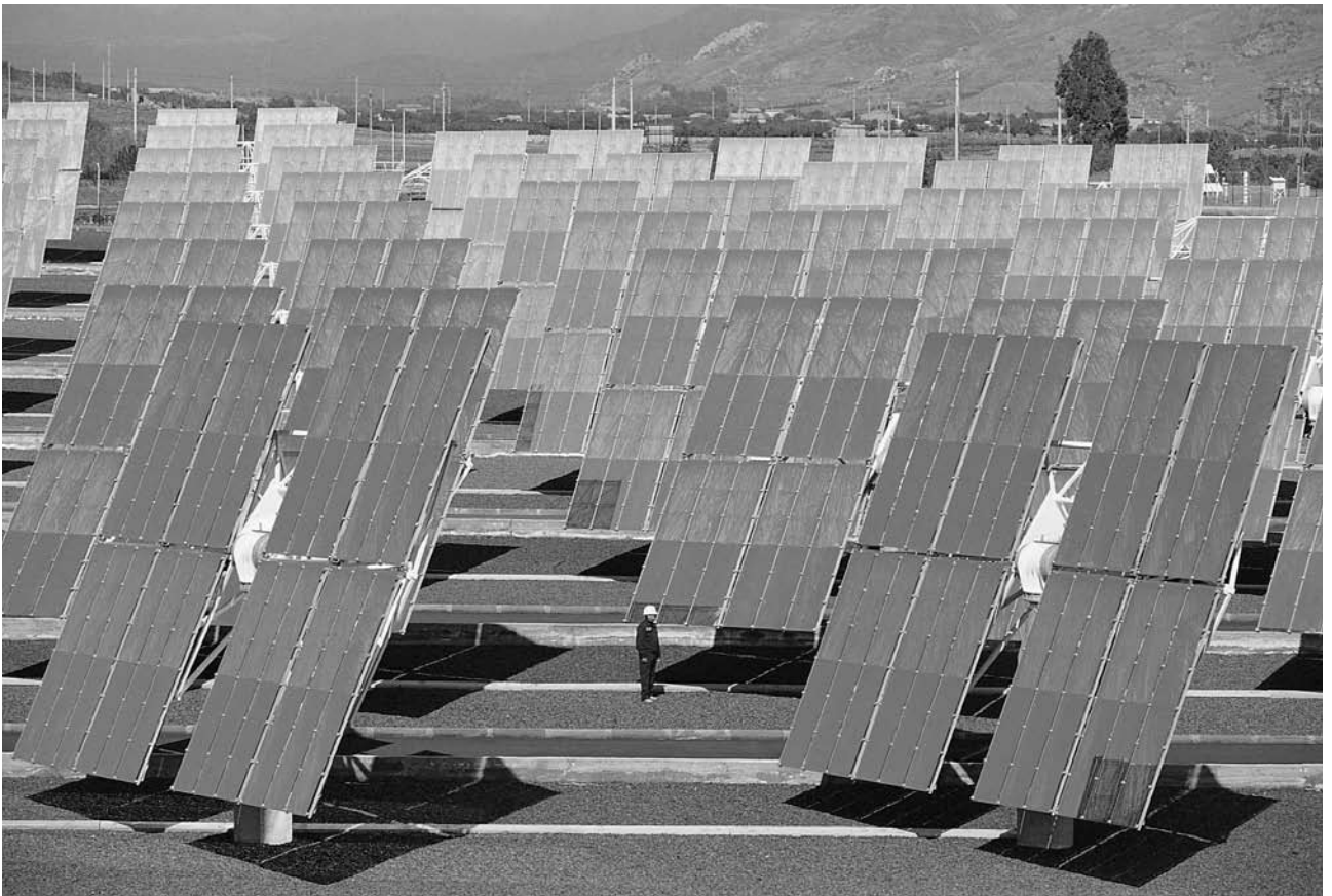
Plate 92 Centrale Solare Eurelios, an experimental solar power plant outside Adrano, Sicily. The continual rise in energy consumption has made the search for renewable forms increasingly important (Photo © DeA Picture Library).
