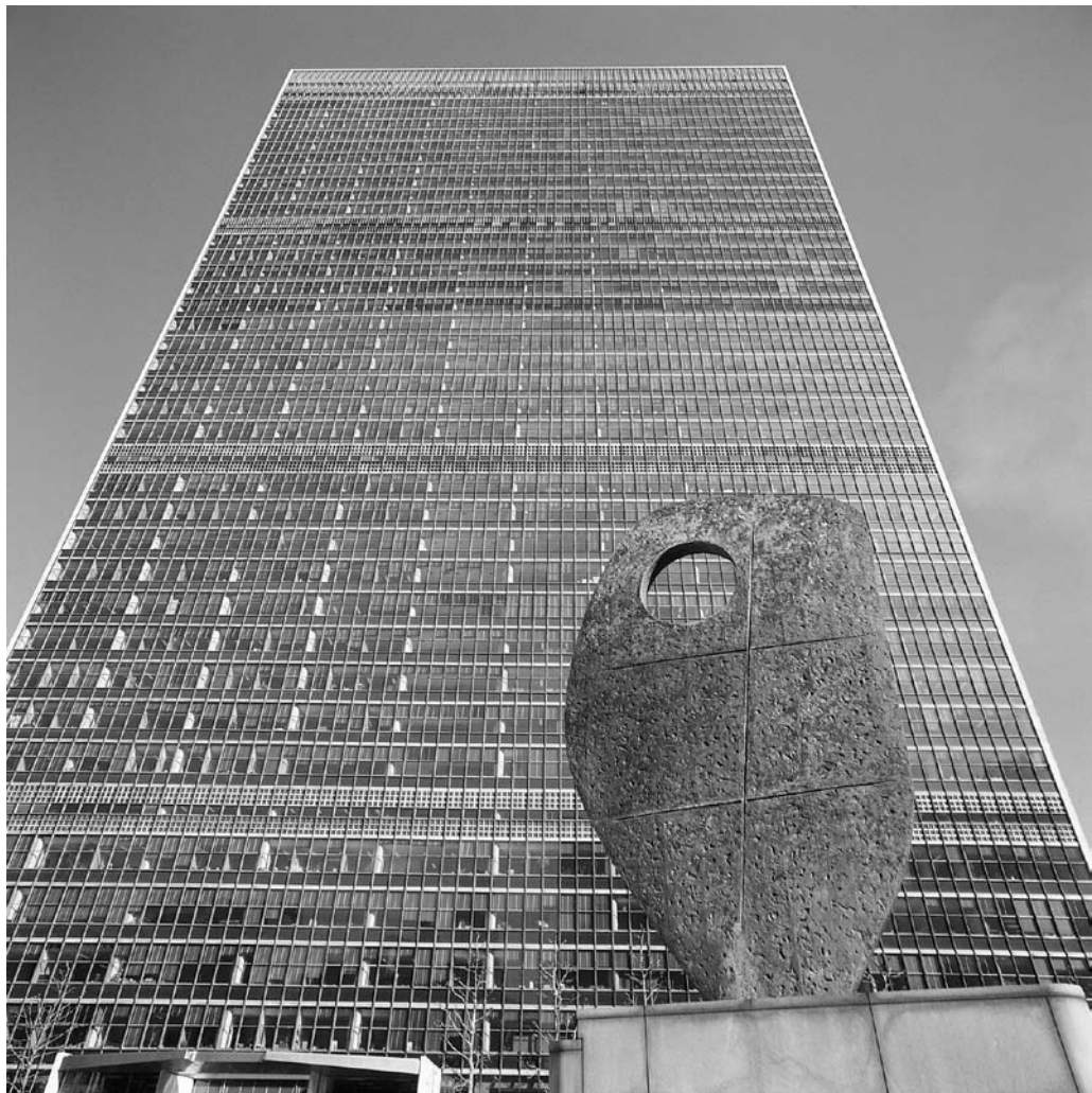
Plate 11 The 39-storey Secretariat building, part of the United Nations Headquarters in New York City, designed by Wallace Harrison with Le Corbusier and others. The UN, the largest and most representative international organization in the modern world, was founded in San Francisco in 1945 (Photo © DeA Picture Library).
