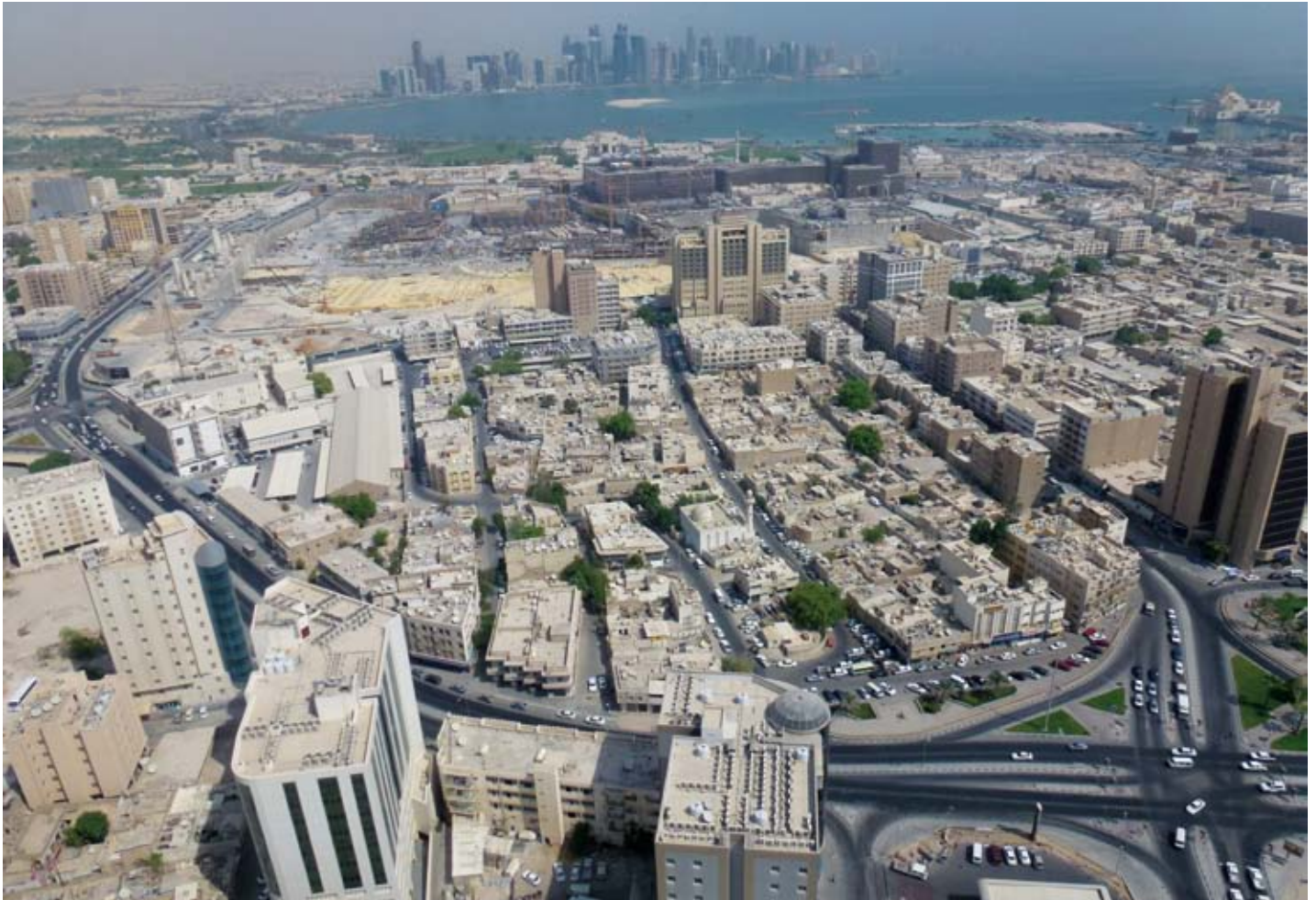
Helicopter view of the heart of Doha. In the foreground are the quarters of Al Asmkah and Msheireb and in the background the modern Diplomatic Area.
