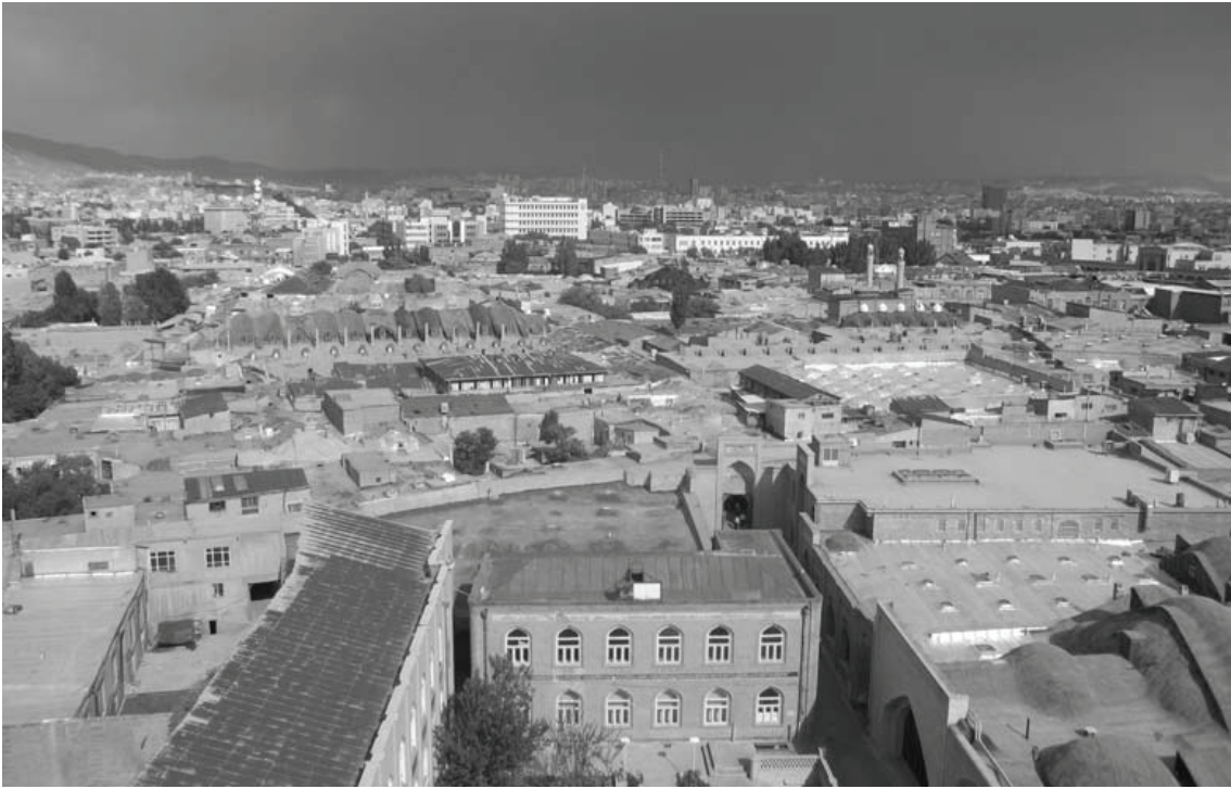
General view of the nominated property
