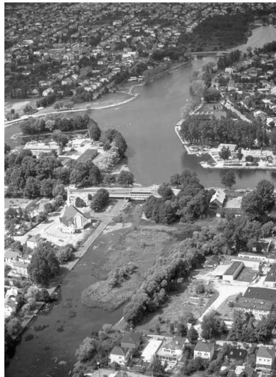
Hydraulic facilities in Augustów
