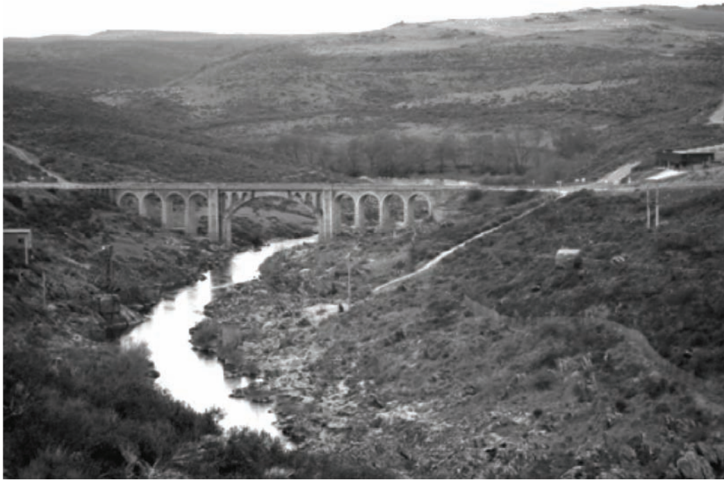
General view of the nominated property
