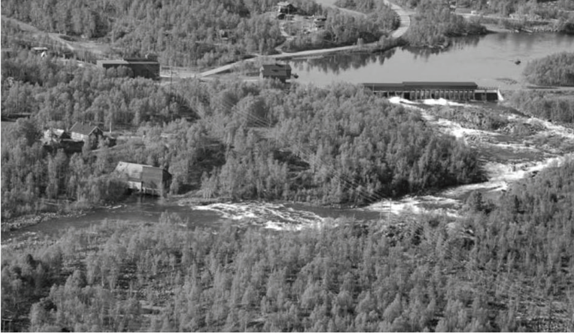
Kuráfossen power station
