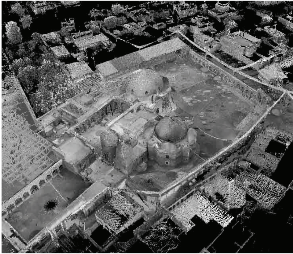
General view of the nominated property
