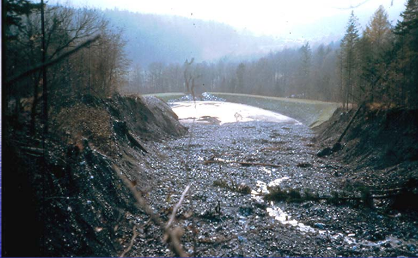
Bank failure collapse
