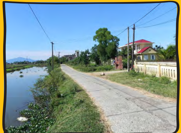
The picture above shows that a road in front of the school is not safe because there is a canal next to it without any protective bars or fence. In the event of flooding, there are no guide posts on the road to distinguish the river from the road itself.
