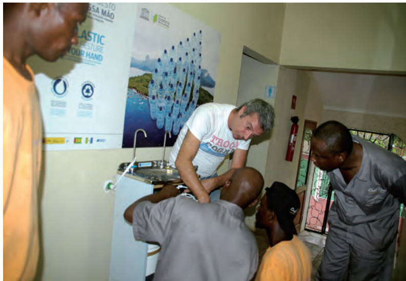
Fig 6. Installation and training of local technicians on the water purifying machines
