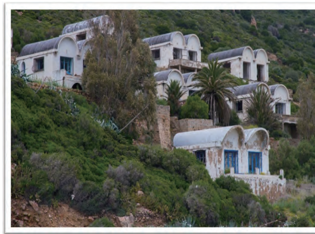
Bungalows existing restore
