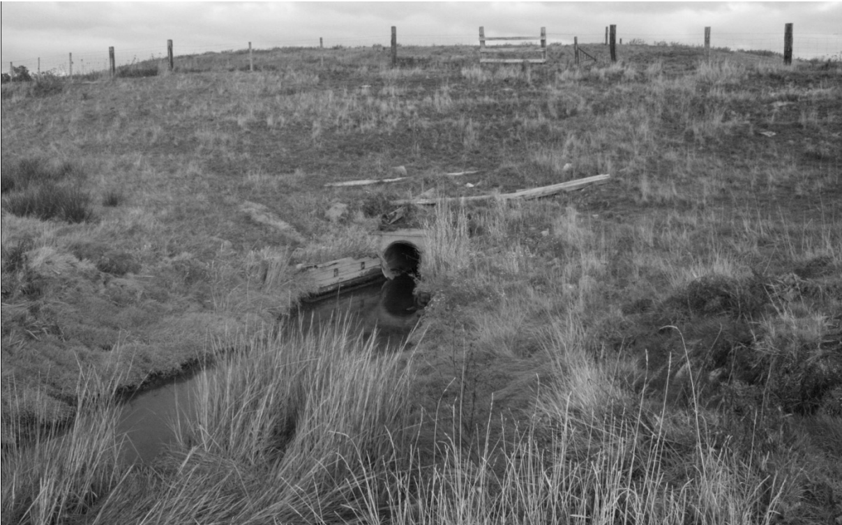
Aboiteau of the drainage system
