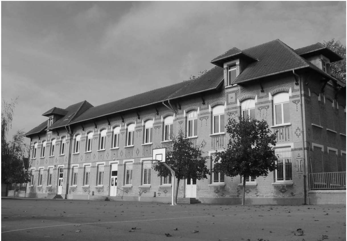
Liévin coal-mining company – school of estate n°16 in Liévin
