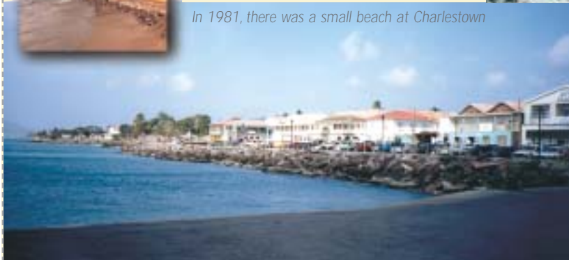
By 2000, the beach had disappeared and land has been reclaimed and protected with a boulder revetment
