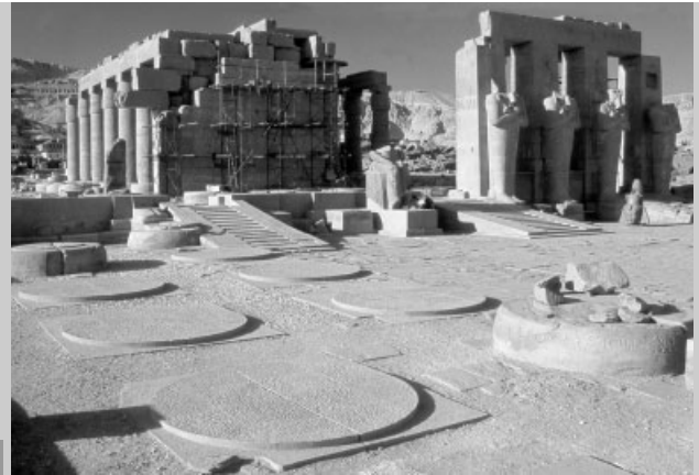
28. Restitution of the bases of Ramesseum's columns, an example of reversibility in restoration, facilitating a better legibility of the ancient temple's architecture.
