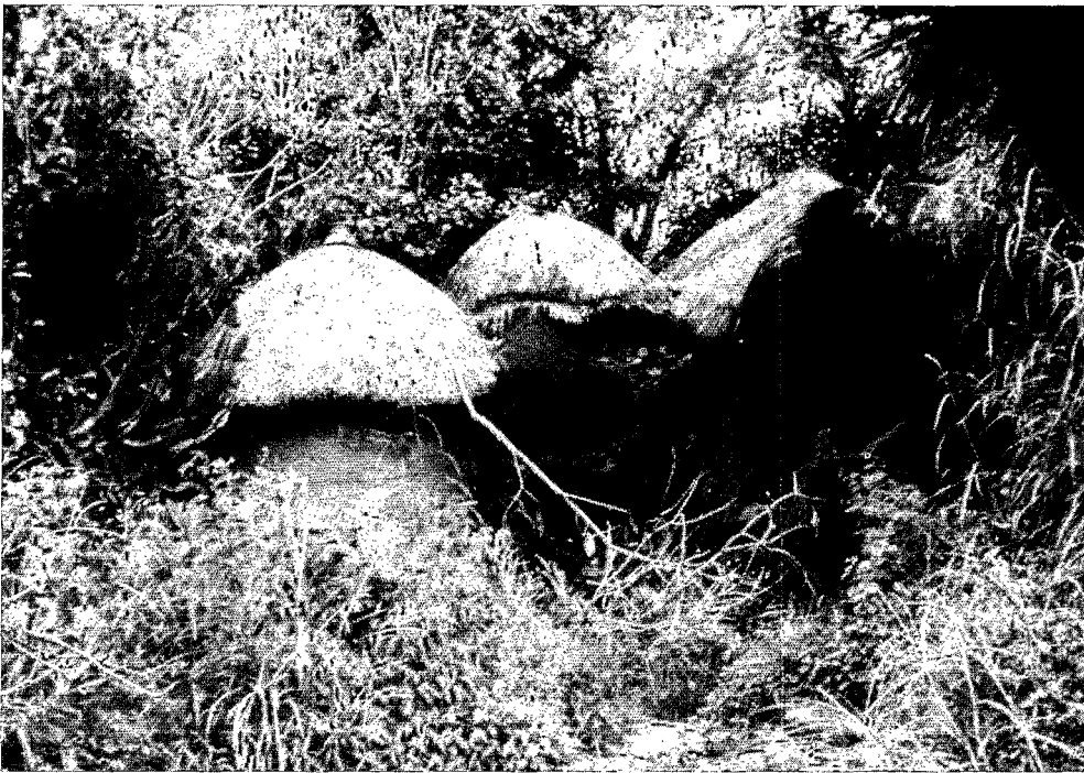
64. PRESERVATION OF THE CULTURAL HERITAGE IN TROPICAL AFRICA. Plateau Province, Nigeria, village of Sha. The village was abandoned towards 1962. The dwellings, no longer kept in repair, are being gradually reduced to a heap of earth. Group of houses, including one which has partly collapsed.
