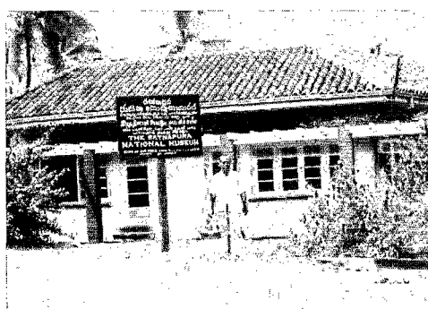
5. NATIONAL MUSEUM, Ratnapura. Vue du bâtiment. 5. View of the building.
