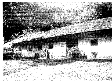
3. NATIONAL MUSEUM, Kandy. Façade. 3. Façade.
