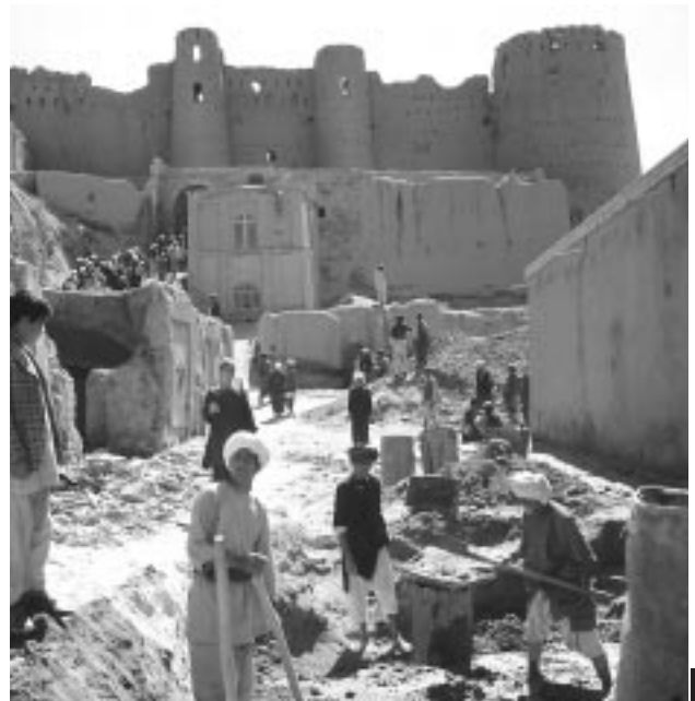
17. Citadel of Ikhtyarrudin, restored by UNESCO from 1974 to 1980 revitalizing traditional skills and the use of traditional materials.
