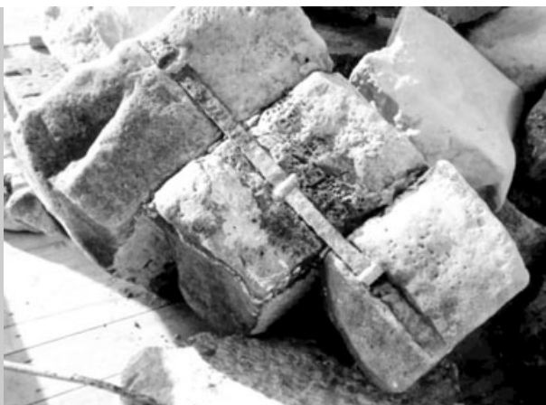
7. The original stones recovered by the SFOR's Hungarian Engineer Contingent (HEC), damaged by bullets and water.
