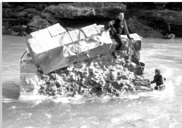
7. The original stones recovered by the SFOR's Hungarian Engineer Contingent (HEC), damaged by bullets and water.
