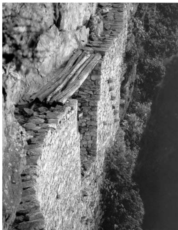
36. A bridge on the Great Inca Route, Machu Picchu, Peru.
