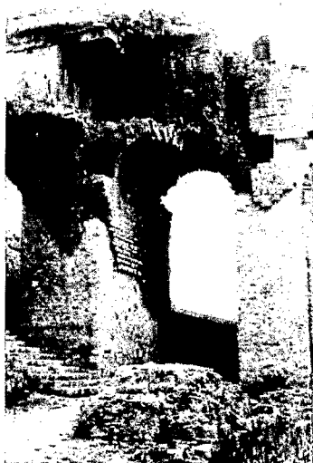
57. The condition of the ruins of Sagunto outside Valencia is deplorable.
