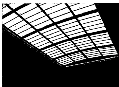
28. MUSEUM VOOR SCHONE KUNSTEN, Ghent. The same glass ceiling, transformed since the war. The putty jointings have been removed and there are fewer armatures. Thermolux laylight.
