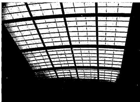
27. MUSEUM VOOR SCHONE KUNSTEN, Ghent. Glass ceiling, pre-war condition. Notice the many putty jointings and the ultra-transparency of the glass.
