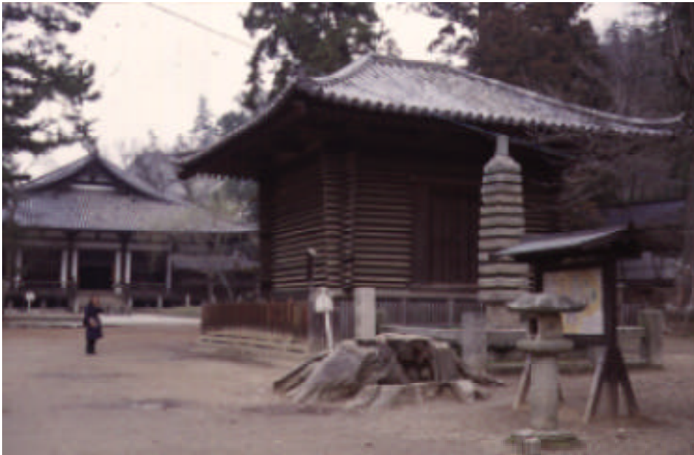
The seventh-century Shosoin treasure house in azekura (log-cabin) style contains relics of the reign of Emperor Shomu, in Nara, Japan.
