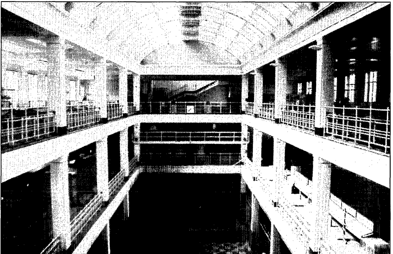
The atrium before reconstruction.
