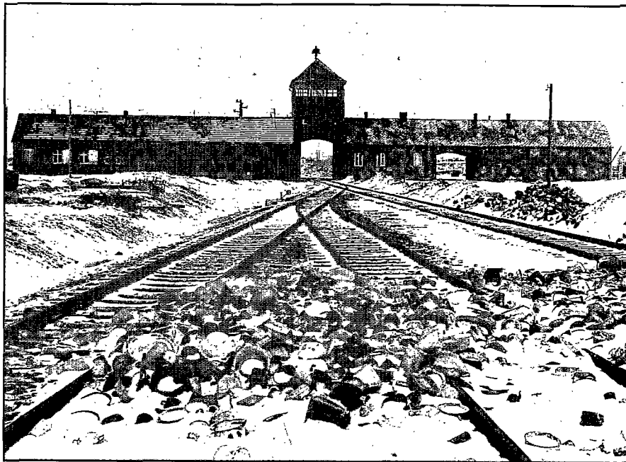
Main entrance gate to the Birkenau camp and a part of the siding.
