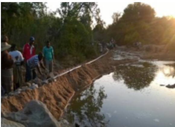
Putting the infiltration gallery in place (Swaziland) Photo: Department of Water Affairs (2014).
