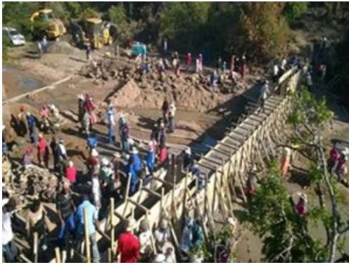
Community involvement in sand dam construction (Swaziland).
