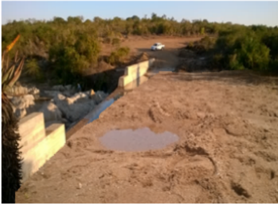
A mature sand dam (of Swaziland)
