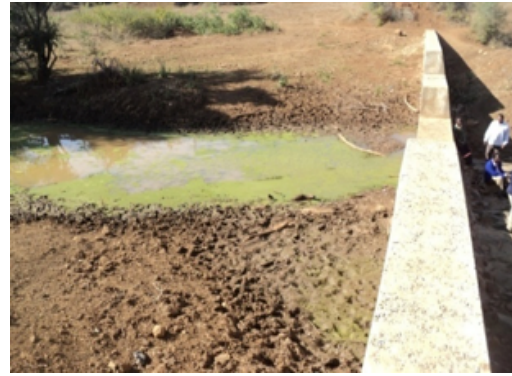
Stagnant water at a maturing sand dam (Swaziland)
