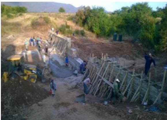
Construction of a sand dam (Swaziland) Photo: Department of Water Affairs (2014).
