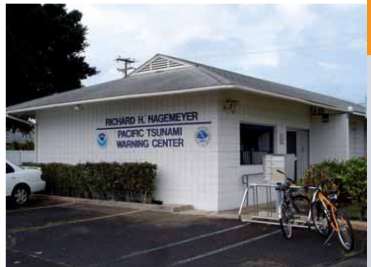
PTWC facilities located at Ewa Beach, Hawaii, USA
