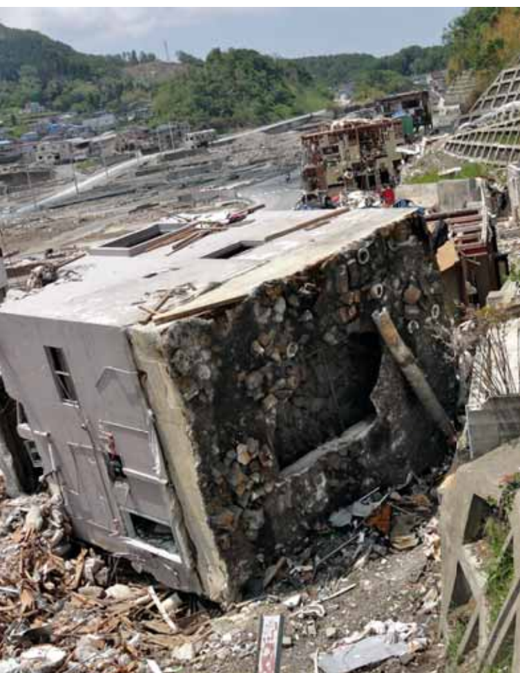
Tsunami flow depths exceeding 10 m and flow velocities over 6 m/s overturned and dragged 3-story buildings as much as 50 m during the 11 March 2011 Japan tsunami. Onagawa, Japan. Photo courtesy of ITIC.
