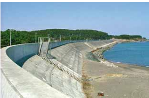
Sea wall with stairway evacuation route used to protect a coastal town against tsunami inundation in Japan. Photo courtesy of River Bureau, Ministry of Land, Infrastructure and Transport, Japan.
