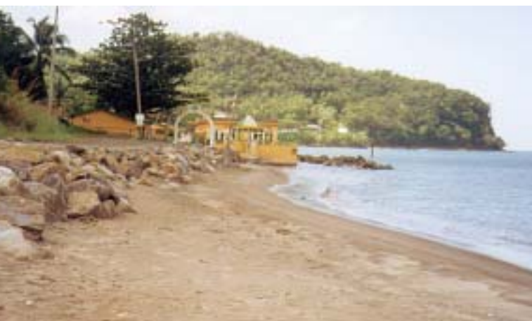
Coconut Beach Hotel, Picard Beach, Dominica in 2000. The hotel was reconstructed after the hurricanes, in the same position. The shoreline has retreated landwards several metres.
