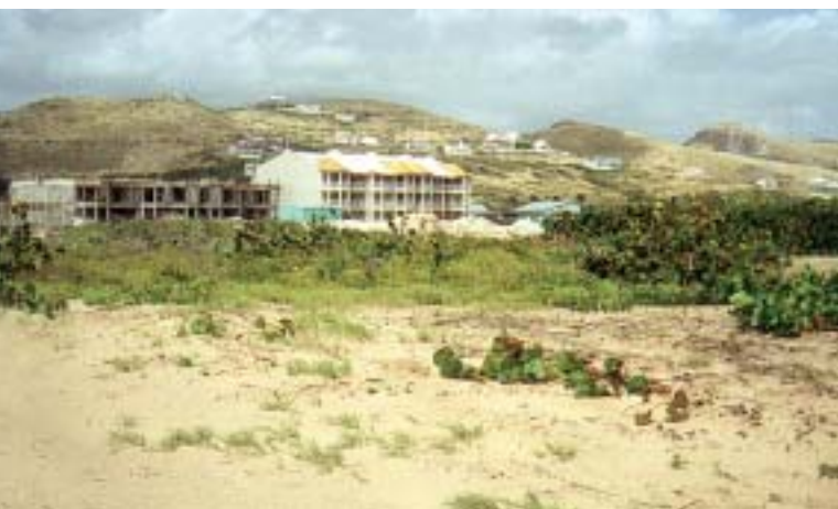
New hotel under construction at Frigate Bay, St Kitts, 2000, well inland from the active beach zone and the seaward dune – an example of good stewardship.
