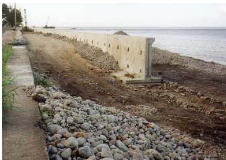
New seawall under construction, Pottersville, Dominica. 2001.
