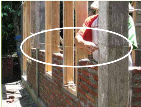
Figure 3.2.20. Laying work of bricks with taut line
