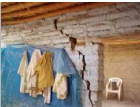
Figure A.2.9 walls of an adobe house, House B
