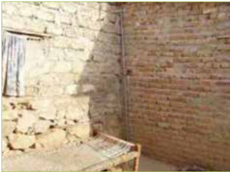
Figure 3.1.22. A house made of various materials of natural stone (lower left), dressed stone (upper left) and bricks (right)
