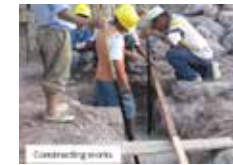
Constructing works Training program in Peru
