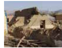
Adobe houses destroyed by Pisco EQ 2007
