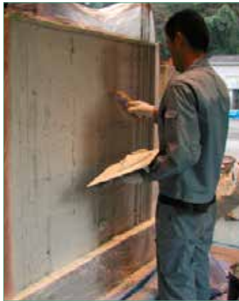
Figure 1. Construction of reinforced PCM wall
