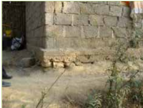
Figure 3.1.23. A house made of solid concrete blocks
