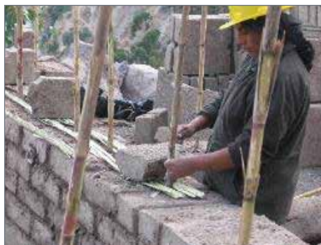
Fig. A.2.4 Installation of horizontal reinforcement from crushed cane
