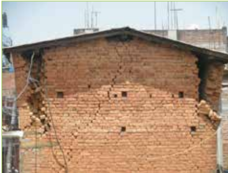
Figure 3.1.8. Damages to RC-framed brick building (Sindhupalchowk District)
