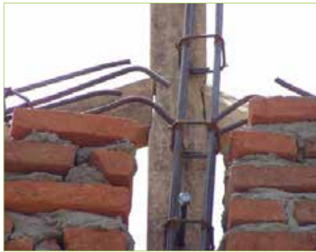
Figure 3.2.6. Construction practice on site Insufficient connection of longitudinal rebar
