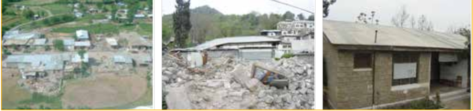
Figure 4.1.1. Small town in mountainous area (left), damaged light roof building (middle) and light roof brick masonry house (right)
