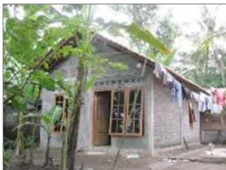
A.2.12 Typical image of reconstructed house
