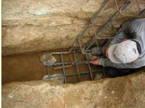
Figure 3.2.10. Excavation works for foundation
