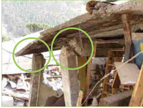
Figure 3.2.6. Construction practice on site Insufficient connection of longitudinal rebar
