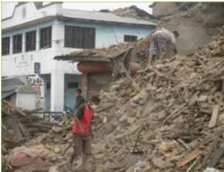
Figure 3.1.1. Completed destroyed structure (Gorkha earthquake in 2015)
