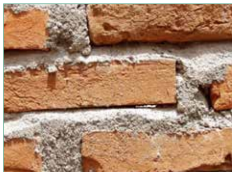
Figure 1.1.8 Bricks eroded by rain (left), and cement mortar with void going through a brick wall (right), in Banda Aceh, Indonesia
