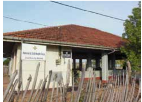
Community center provided by the Government of Japan in Iqbal Nagar, Kuchchaveli, Trincomalee, Sri Lanka (Photo: July 2015)
