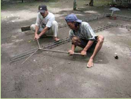
Figure 3.2.17. Bending works of rebar on ground with simple tools without machines
