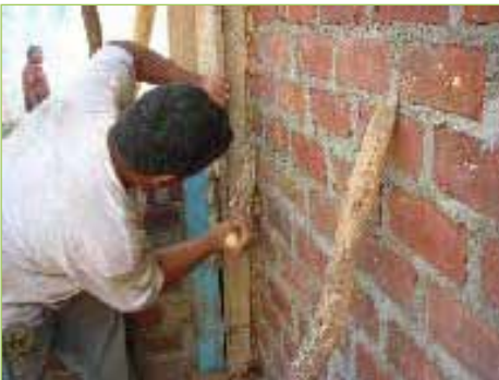
Figure 3.2.13. Form works Packing of small piece of cement bags is usually
