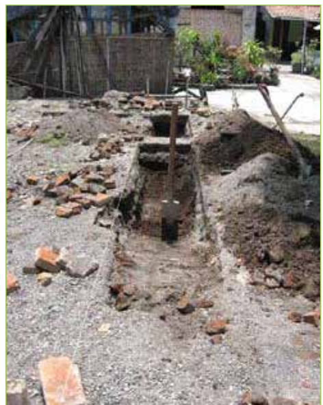
Figure 3.2.16. Excavation works for foundation
