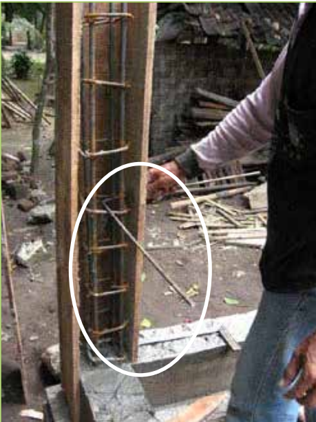
Figure 3.2.19. Anchorage of walls to column
