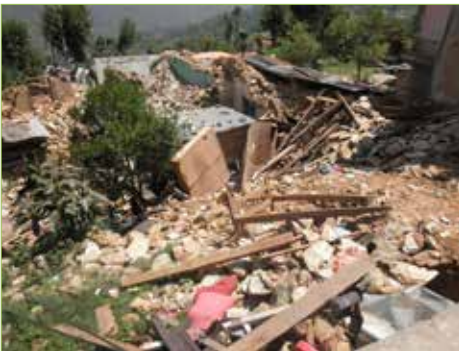
Figure 3.1.3. Damages of houses (Sindhupalchowk Districts)
