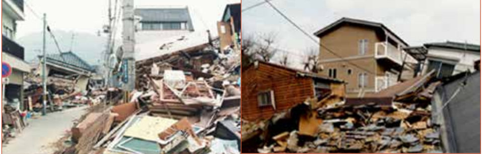
Figure 5.4.3 Many wooden houses collapsed in the Kobe Earthquake 1995 (left), but new houses, following the revised code in 1981, suffered little damage, even in otherwise heavily damaged areas (right)
