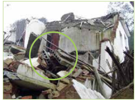
Figure 3.1.15. The same building as in Figure 3.1.14. (Hollow core slabs were observed)
