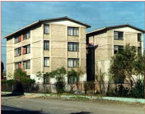
Figure 5.2.8 A confined block masonry building in Chile. From a report by Moroni, O. Gomez, C and Astroza, M.
