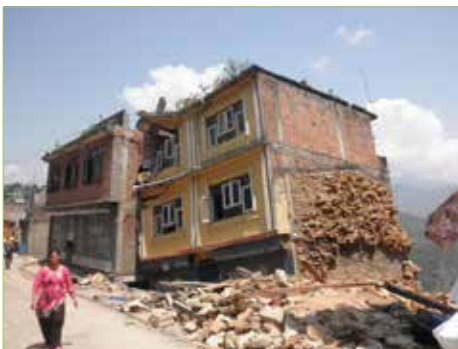
Figure 3.1.8. Damages to RC-framed brick building (Sindhupalchowk District)
