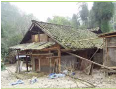
Figure 3.1.16. Timber house that did not collapse
