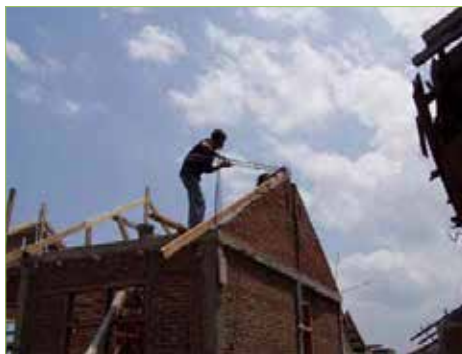
Figure 3.2.8. Placing the assembled rebar of a roof beam fabricated on ground
