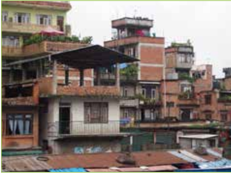
Figure 3.1.4. RC frame with masonry infill walls in urban area
