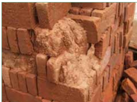
Figure 1.1.8 Bricks eroded by rain (left), and cement mortar with void going through a brick wall (right), in Banda Aceh, Indonesia
