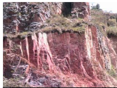
Sandstone to infiltration of water
