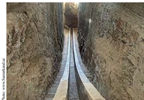
The main instrument of the Ulugh Beg observatory was a meridian quadrant arc with 40 m radius. Its excavated remains are open to the public
