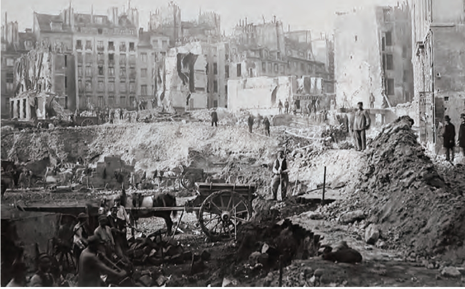
Major urban transformation works of Baron Haussmann on the Avenue de l'Opéra, Paris (France) © Charles Marville, 1862. Source: gallica.bnf.fr - Ecole nationale des ponts et chaussées*
